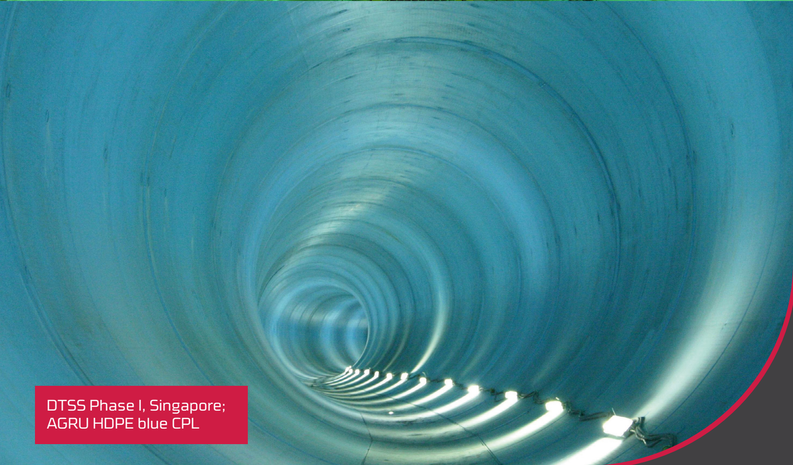
CPL Installation in a Double Shell Tunnel Lining
